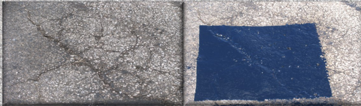
Repair Alligator Area - Raise Low Spots -
